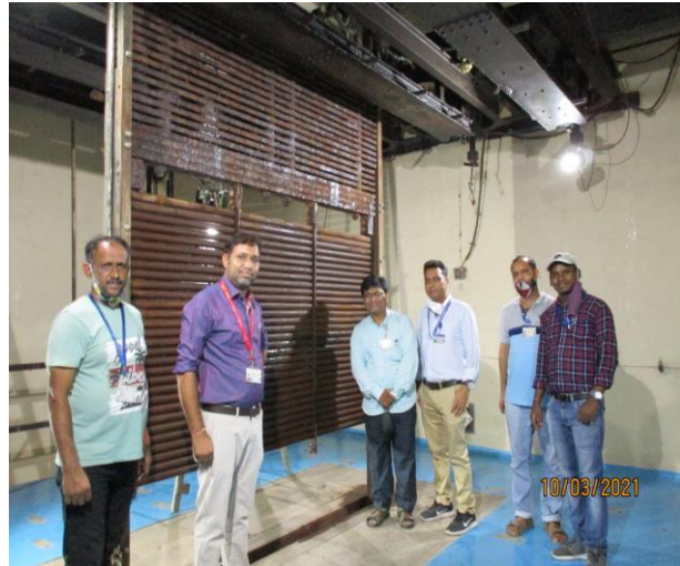
Figure 5: Actual condition of Source Frame after removing all the active Co-60 sources from frame.
