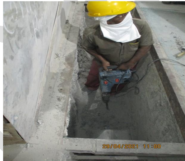
Figure 6: Source Pit excavation work in progress.
